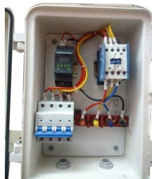
Fig m: polycarbonate junction box with bus bar arrangement and 6 Amps miniature circuit breaker.
